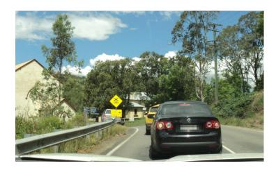
In the 18 months to July 2021, there were four accidents at this site, mainly as a result of approaching vehicles being unaware of the vehicles queued at the level crossing beyond the crest. In one case, the vehicle involved became airborne and ended up against the wall of the adjacent former court house. The consequences of a loaded quarry truck being involved in an accident with the queue are potentially fatal.
