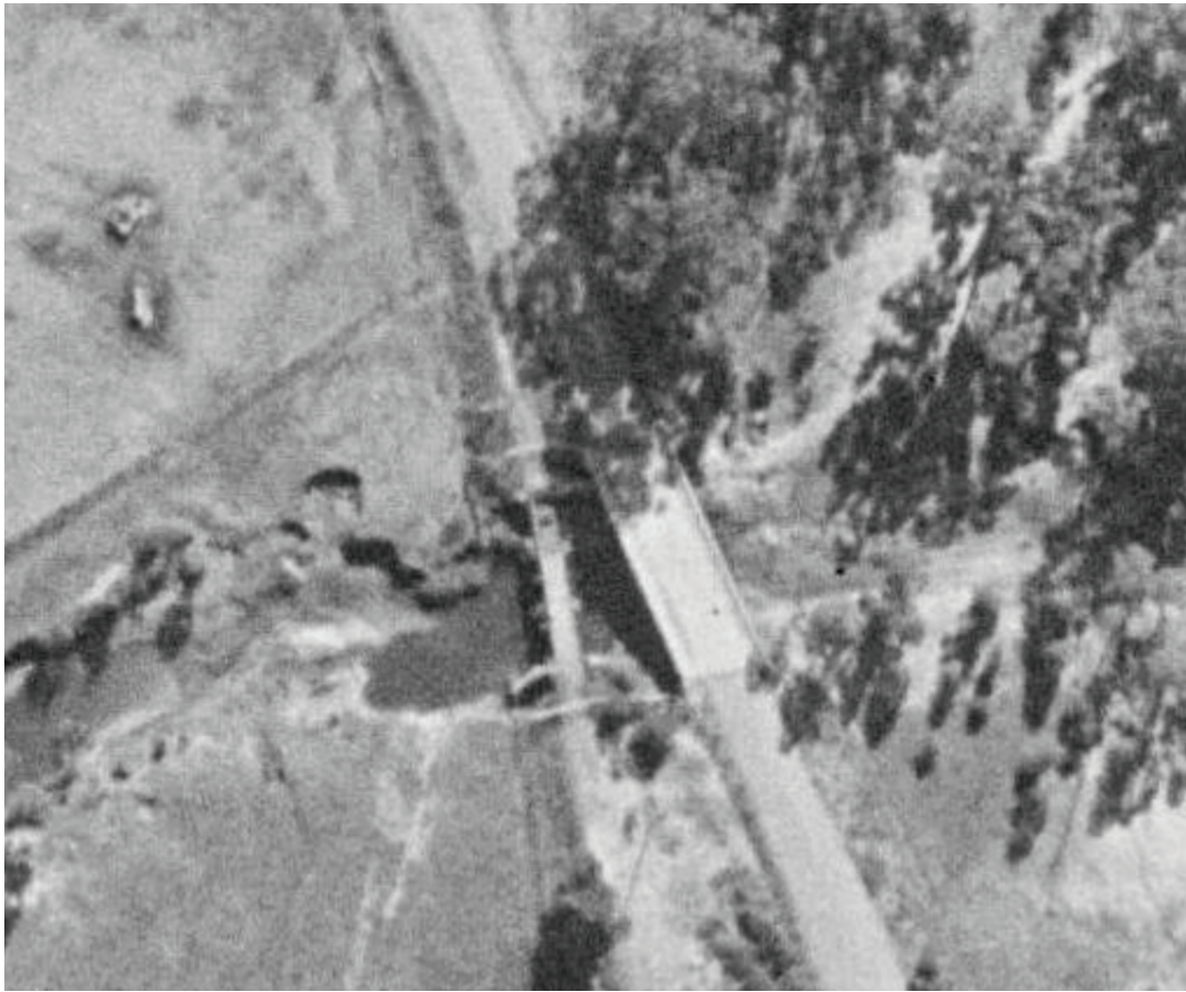
Harris Creek military railway bridge 1943 Aerial Photography SIX NSW Lands Dept
