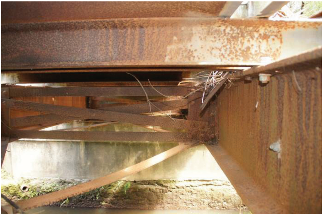
Remaining superstructure under the Bailey bridge span Phil Hurren Jan 2016
