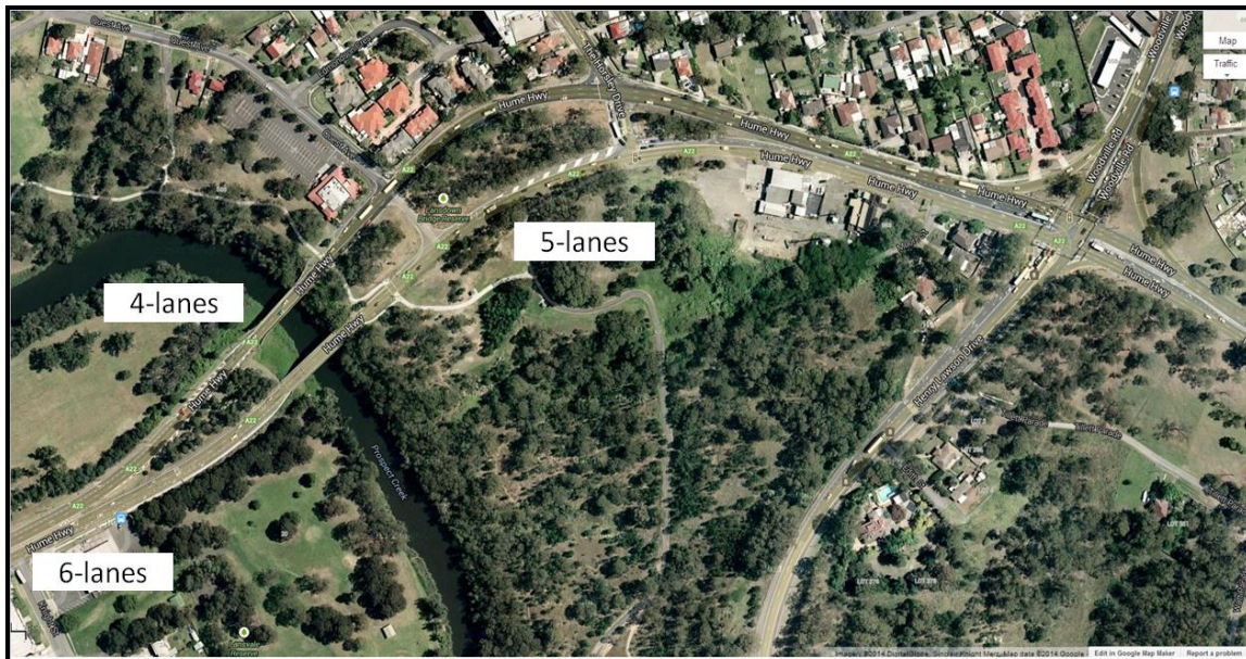
Figure A4 3 2-lane bridges over Prospect Creek
