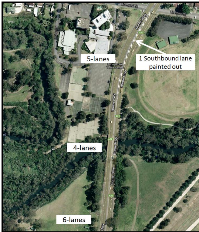
Figure A4 2 4-lane Bridge over Cabramatta Creek
