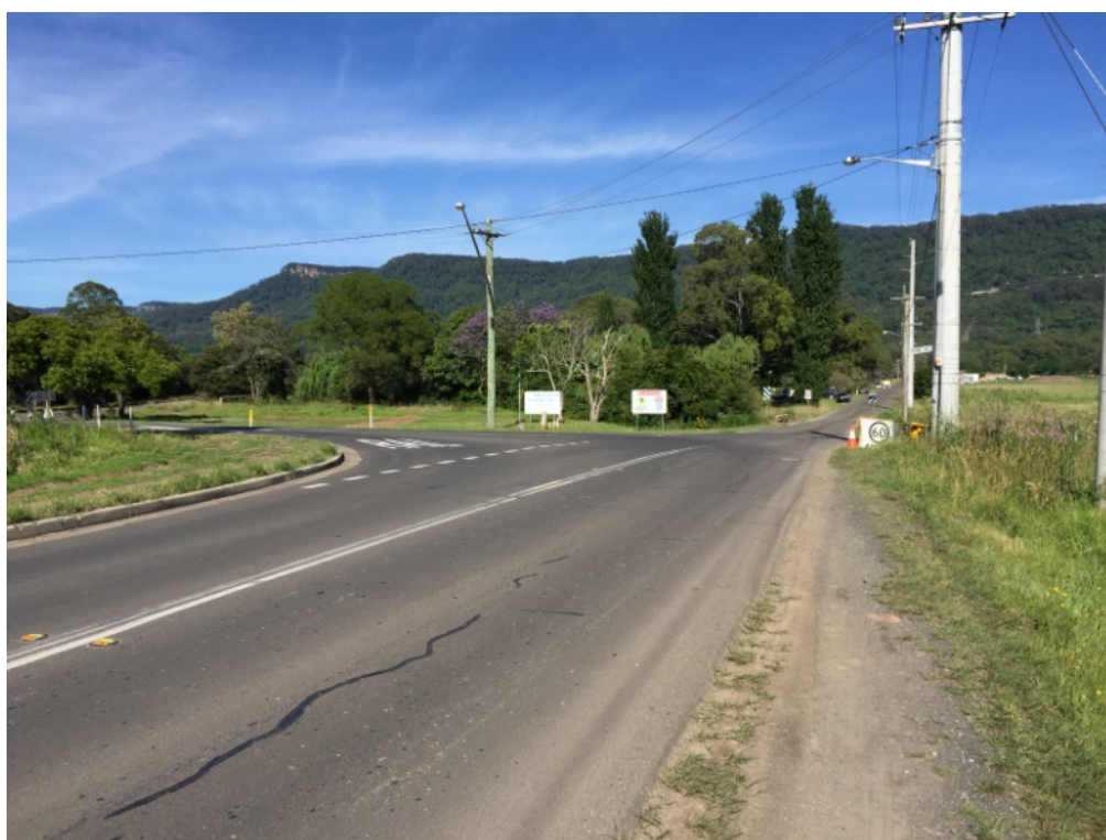
Plate 1 Wongawilli Road & Shone Avenue Intersection Signage
