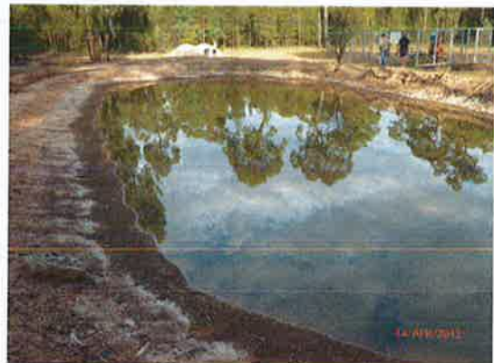
Unlined produced water holding pond
