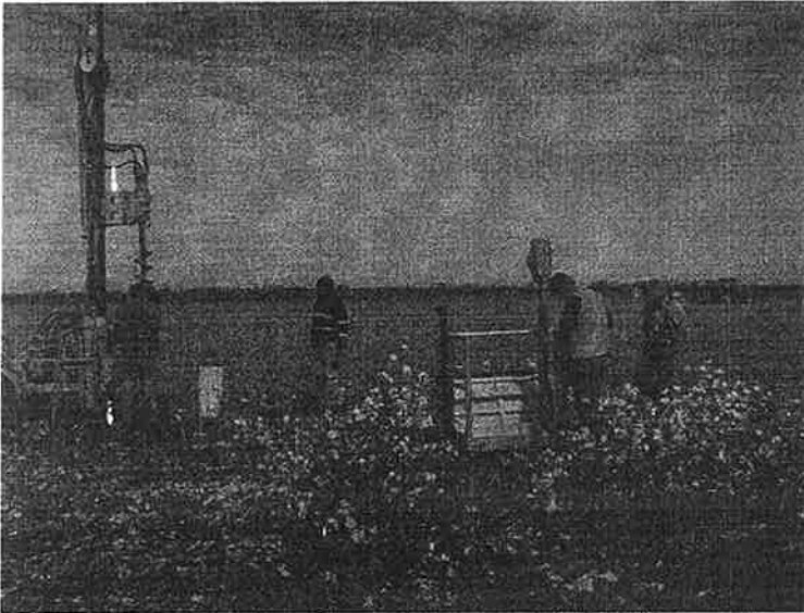
Figure 4 On the left - Grant Millar and (NR&M) installing one of the NR&M barrel lysimeters - close to (on the right) the large (shelve-type) CSIRO lysimeter at ACRI, Narrabri (May 2005). Picture courtesy of Dr. Des McGarry.
