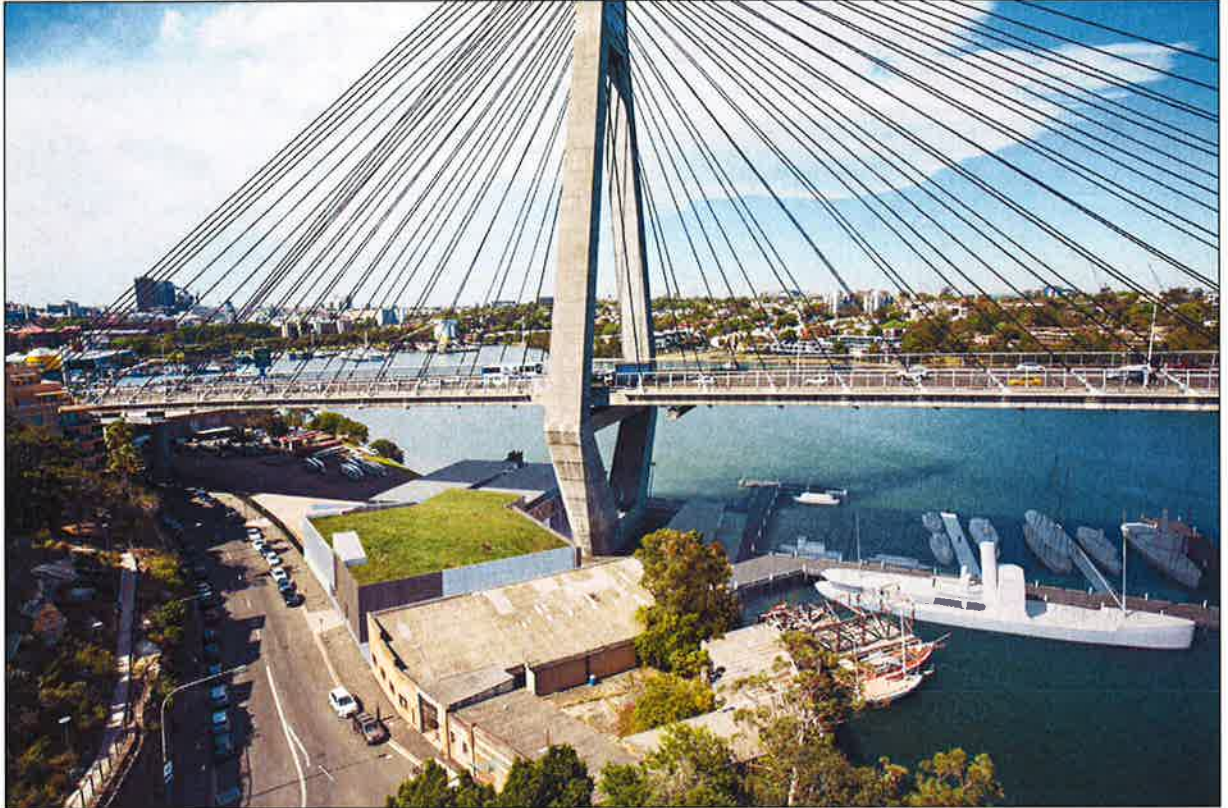
Figure 17: 3D Photomontage of the completed maritime facility, including the Fleet's vessels in their berths (looking south)
