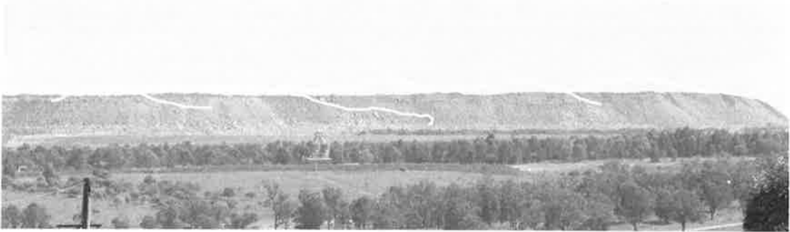
Figure 3.13 | Example of a typical bund with suggested modifications to ridge profile as considered in Workshop One overlaid.
