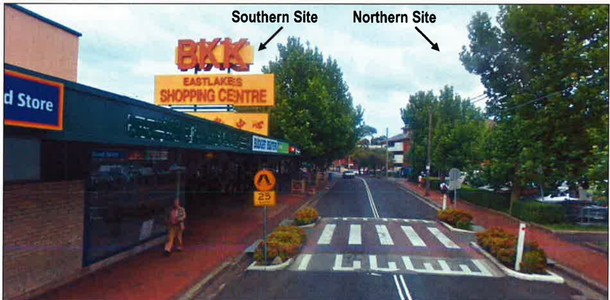
Figure 3: Site as viewed looking west along Evans Avenue (Base image: Google Maps)
