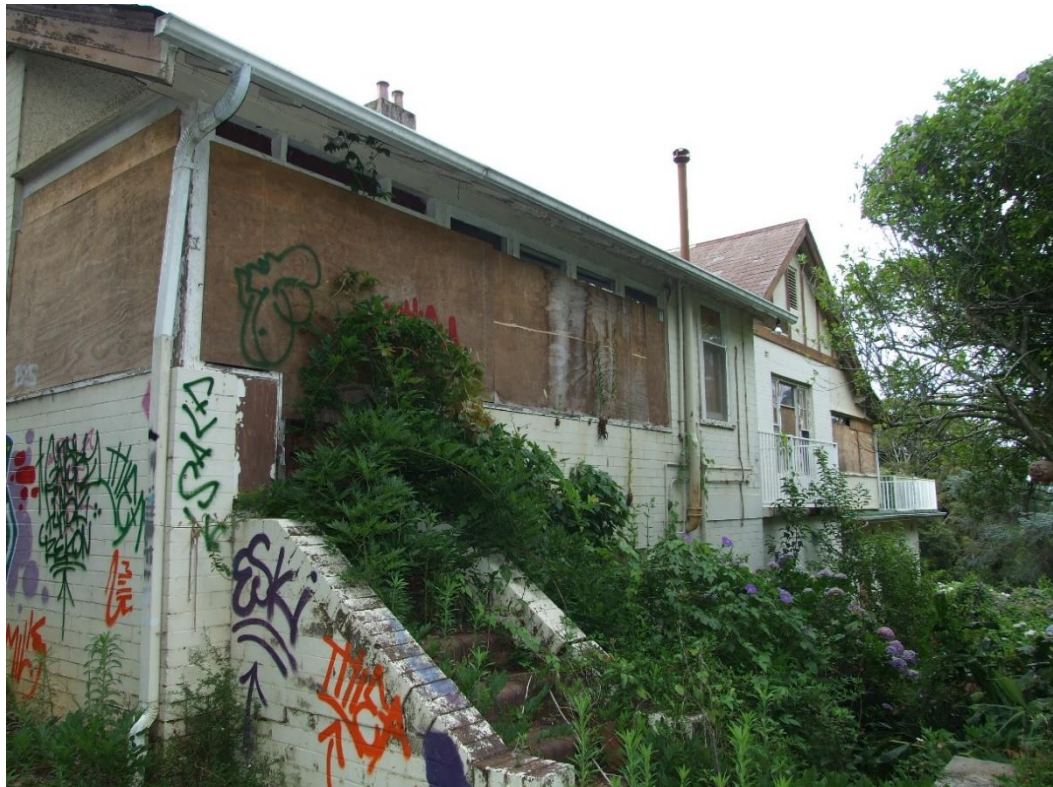
Figure 11 - The rear of the house showing the later enclosed verandah and the extension and Billiard Room Terrace to the south.
