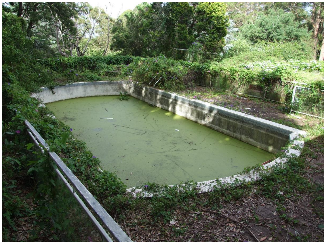
Figure 14 - The modern elevated pool terrace and swimming pool which is proposed to be demolished in this application.
