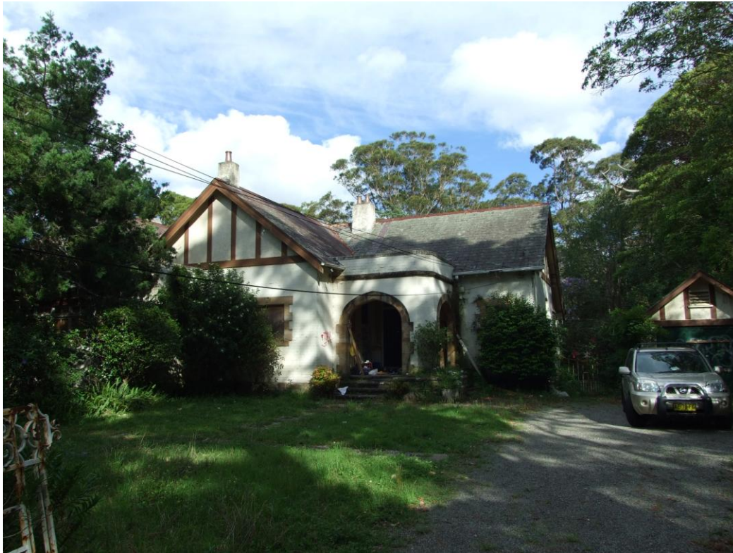
View of No. 1 Avon Road from the entry gates showing later porch and gabled form of original building.
