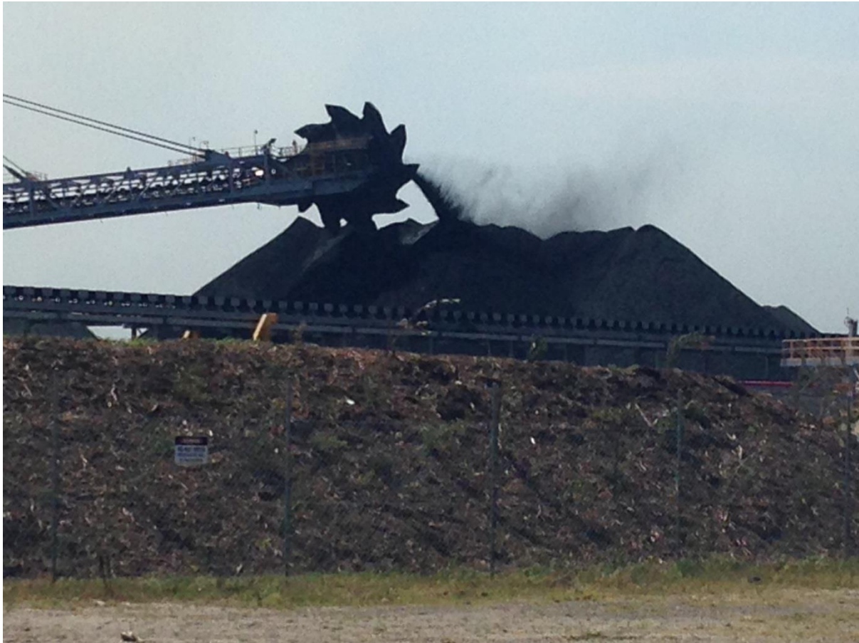
Figure 1: Existing coal loader on Kooragang Island operating on 17 October 2013
