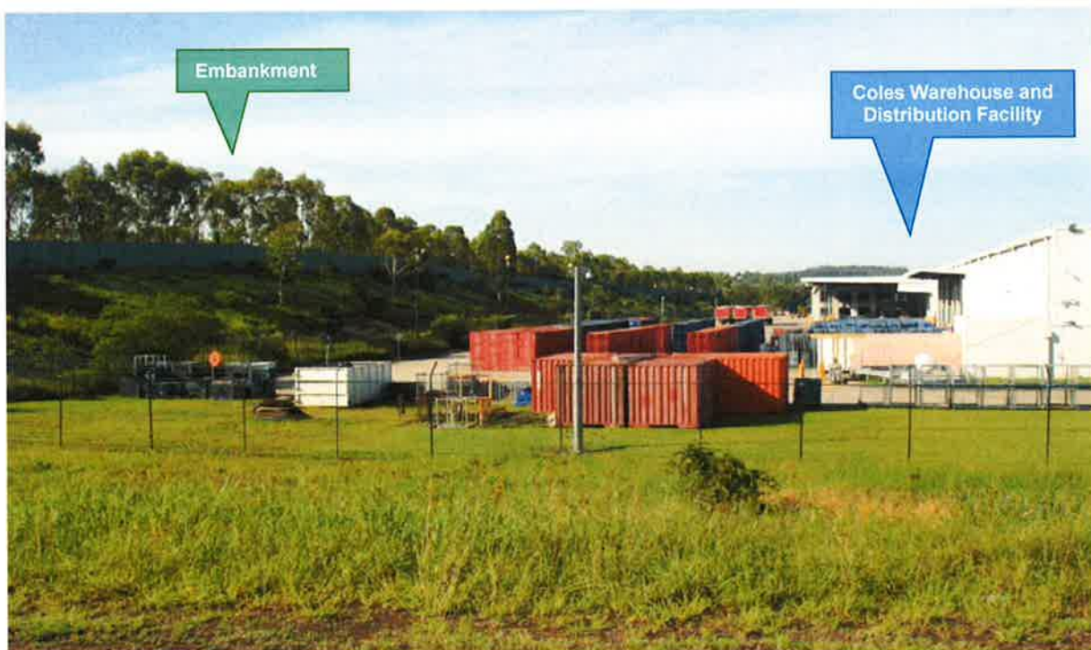
Figure 8: View south-west to rear of adjacent Coles site and the embankment
