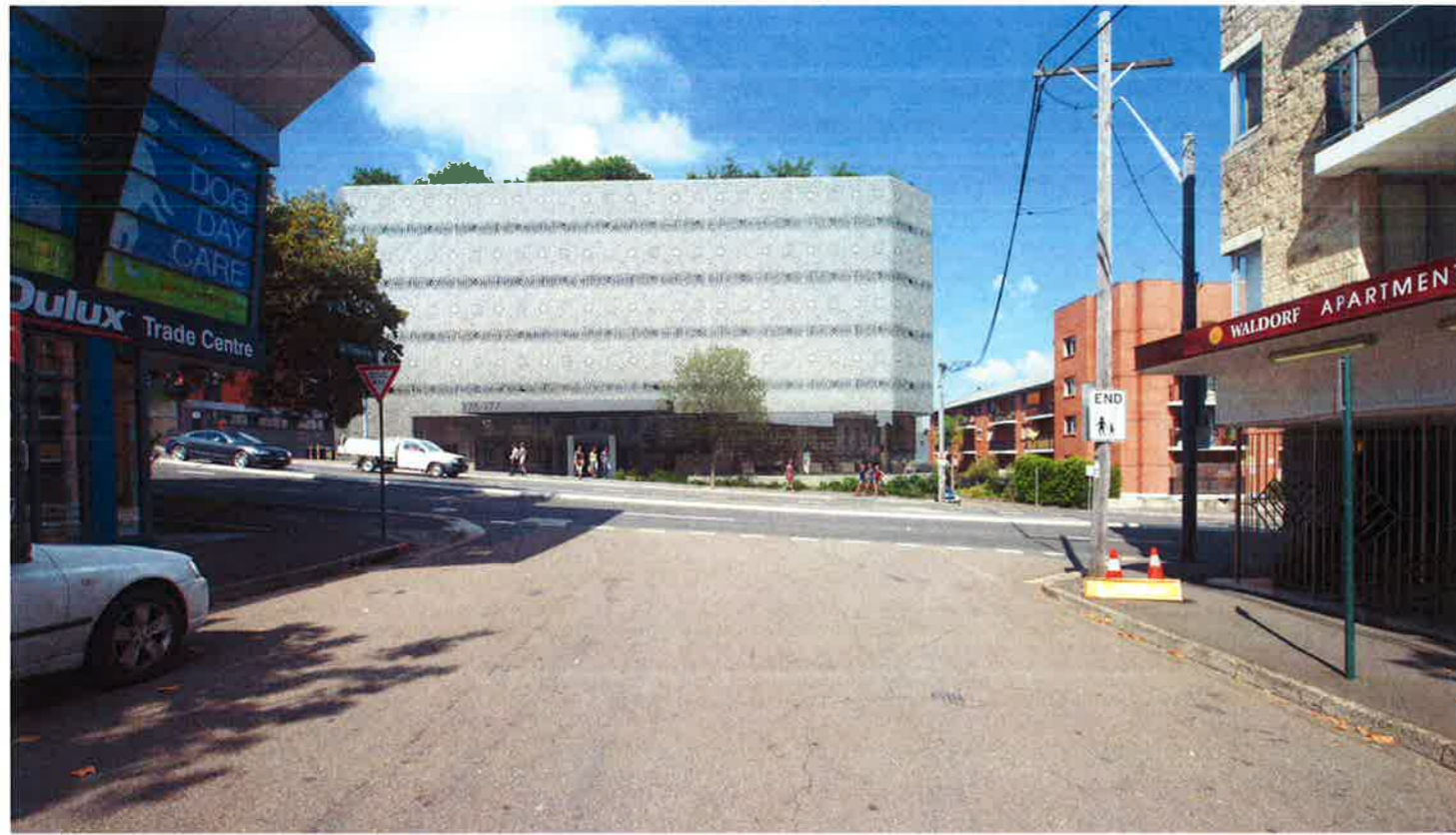
CLEVELAND STREET ELEVATION OF APPROVED DA SOURCE: DEPARTMENT OF PLANNING & ENVIRONMENT WEBSITE SSD 14_6371
