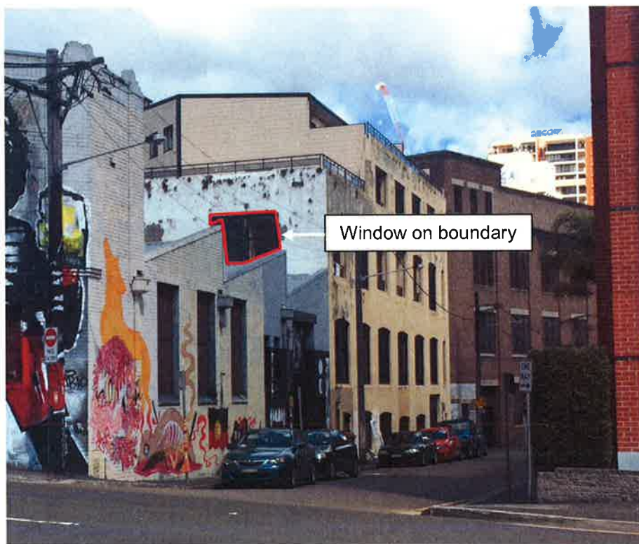
Figure 17: Image showing window of 6-8 Woodburn Street on boundary of subject site.
