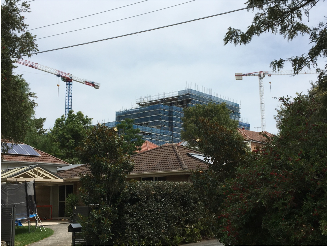
Building on Constitution Rd towering over houses in Richard Johnson Cres
