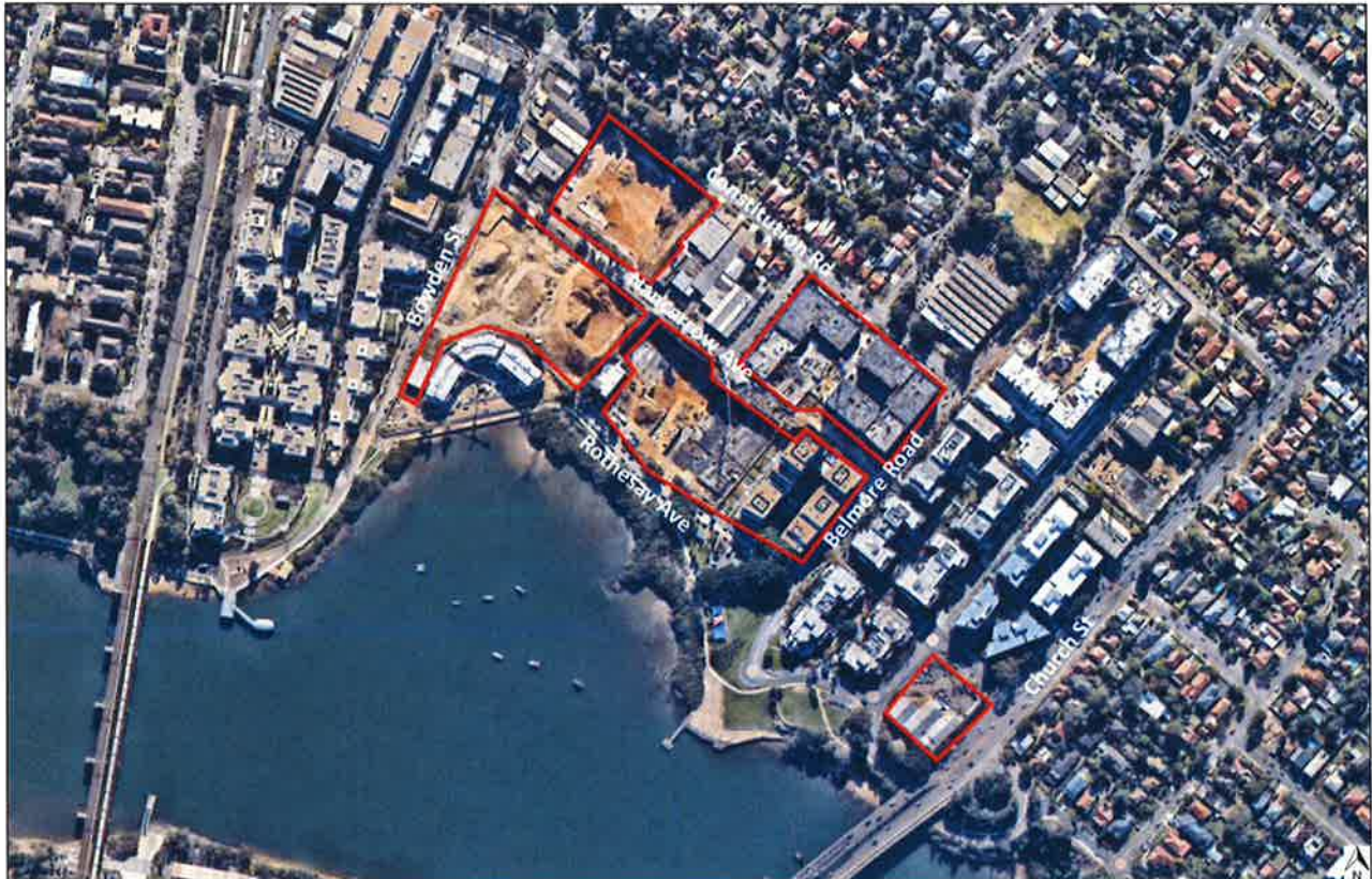
Figure 2: Aerial view of the site indicating current stage of construction works (Base Source: Nearmap)
